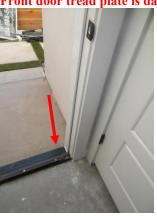
\*\* Weather stripping and front door tread plate repaired by builder prior to closing.
