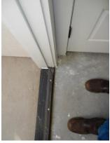
Front door tread plate is damaged
