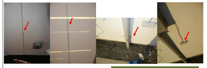
Gap between the stucco base metal drain and the foundation. Protect the substrate
