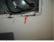
\*\* Gaps and GFCI repaired by builder prior to closing.
