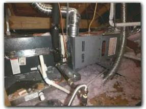
It is recommended that a screen covering be installed at the ceiling of the furnace closet to reduce the risk of insulation falling into the closet and/or rodents from entering the closet.
