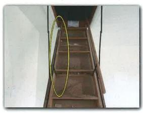
There should be a 2 foot wide floored path from the attic access stairs to the furnace and a/c units in the attic. Additional flooring is needed to cover the void(s) in the existing flooring.
