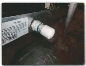
Need to remove the insulation from the drip pan under the a/c units in the attic to reduce the risk of the secondary drain pipe from becoming clogged and allowing water to overflow and penetrate the structure.
