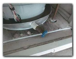
The supply of combustion air (and draft air) for the water heater may be insufficient. When combustion air is required, two openings are normally required. One should be located within the uppermost twelve inches of the enclosure and the other within the lower twelve inches of the enclosure. This condition represents a health hazard that should be further investigated by a Licensed Plumber and repaired as necessary.
