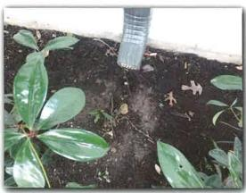
The bottom section of the downspout is missing at the southeast corner.
