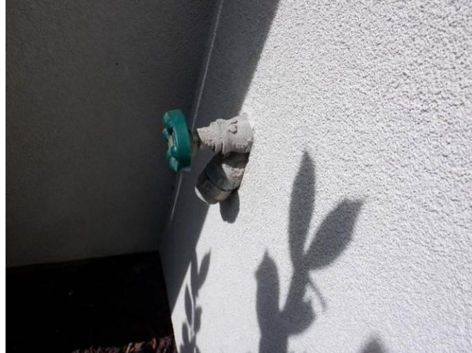
Photo 39: All exterior faucets were embedded into the stucco (east side is shown).
