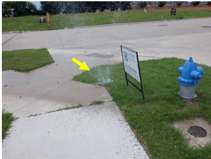
Photo 46: At least one leak was noted at the south end of the parkway.
