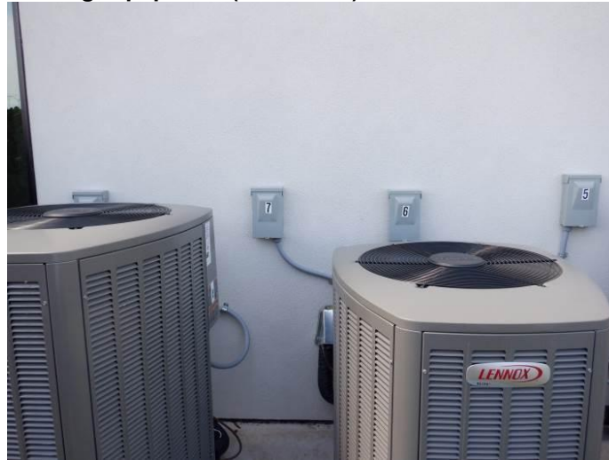
Photo 21: The services disconnect panels for two exterior condensing units were located behind the condensing units.
